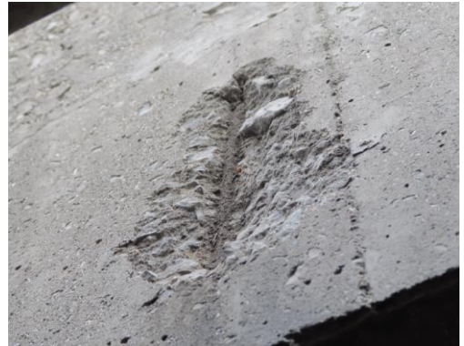
Fig. 9 Visible concrete spalling induced by corroded rebar on lateral surface of deck
