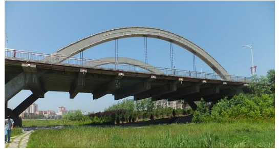
Fig. 8 Landscape of reinforced concrete arch bridge
