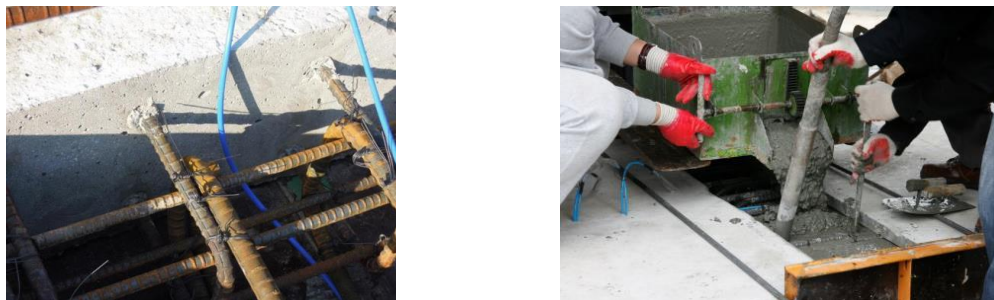
Fig. 4 Casting of high strength concrete in a joint
