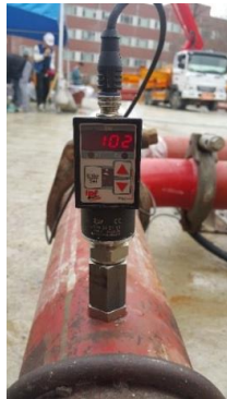
(a) Installation of pressure sensor
