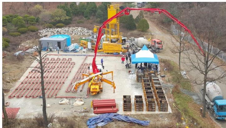
Fig. 7 The whole view of pumping test site
