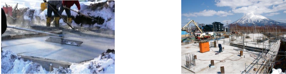
Fig. 1(a) Placement of concrete in cold weather (ACI 2010) (b) Curing of concrete in cold weather (Krylov 2008)
