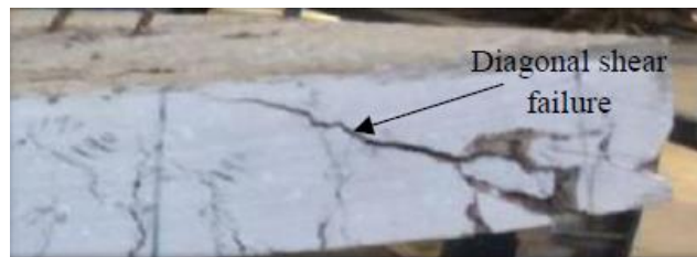
Fig. 22 Mode of failure in slab HS9-B
