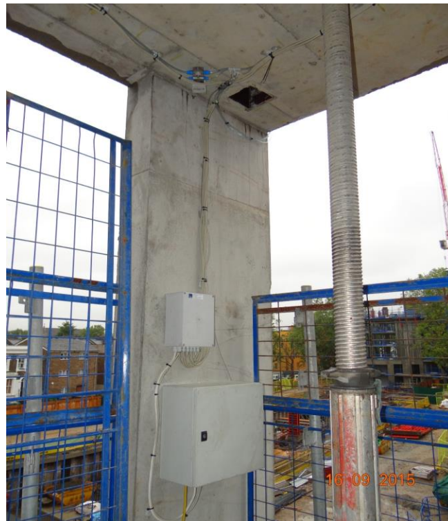
Fig. 5 Hydrostatic cells levelling connected to data box
