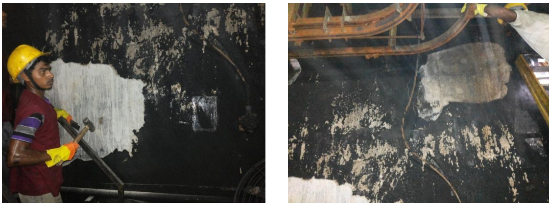
Fig. 2 Dark patches of burnt zones on the interior walls
