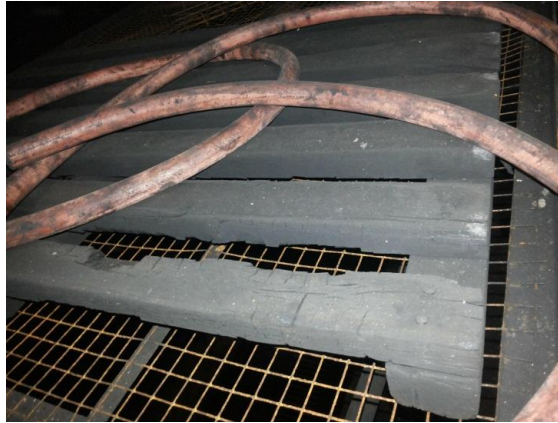
Fig. 3 Burnt wooden frame found in the proximity of the source of the fire
