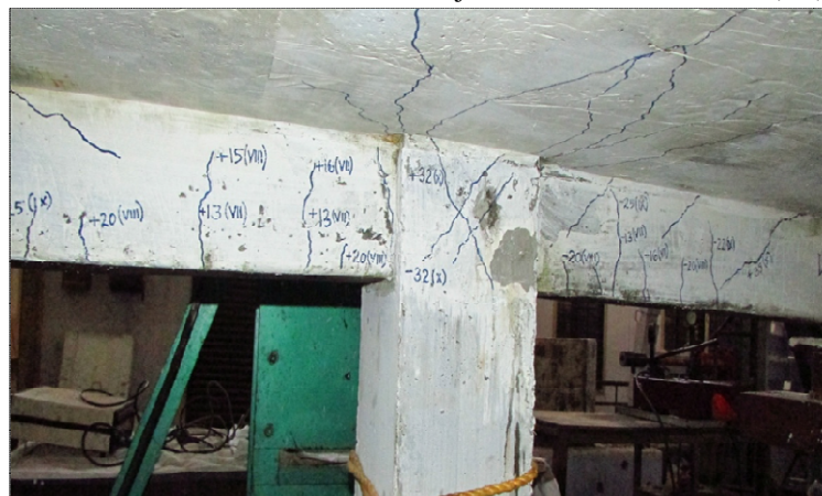
(c) SFRHPC interior beam-column-slab joint with 1.0% steel fibre (A3)
