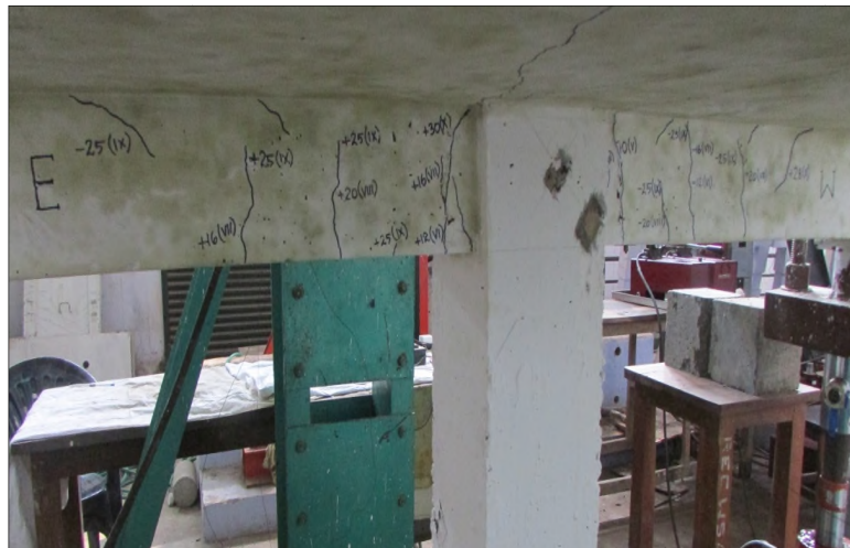
(b) SFRHPC interior beam-column-slab joint with 0.5% steel fibre (A2)
