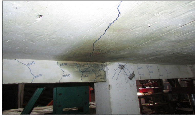
(a) HPC interior beam-column-slab joint (A1)
