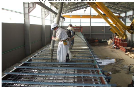
(g) Casting deck slab
