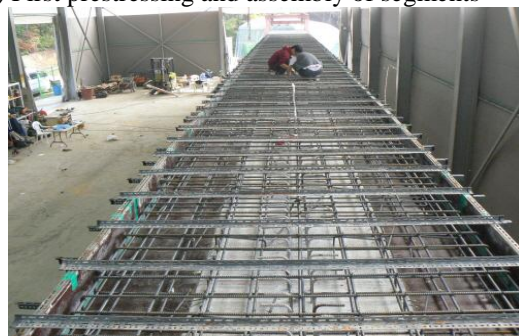
(f) Placing of slab rebars
