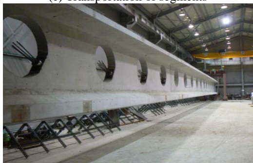
(e) Erection of girder
