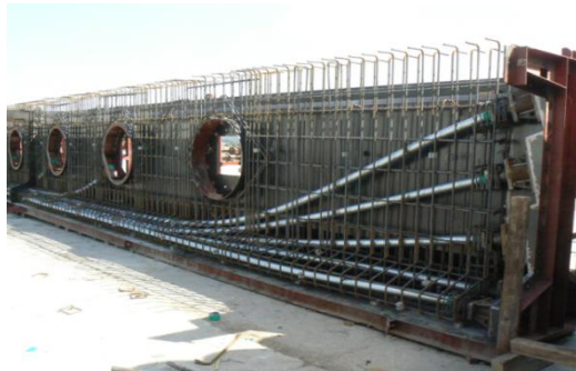
(a) Placing of rebars and ducts
