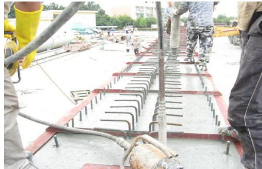
(b) Casting girder concrete
