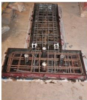
Fig. 3a Reinforcement cage in steel mould
