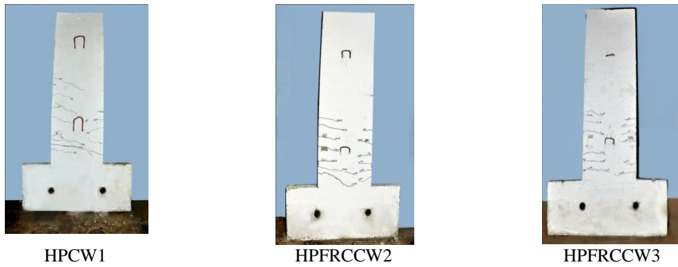
Fig. 6 Crack patterns of HPC and HPFRCC structural walls
