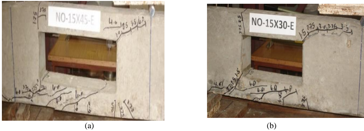
Fig. 5 Shear failure of beam specimens with un-strengthened openings
