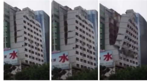
Fig. 4 Collapse with overturning (containing both material nonlinearity and geometric nonlinearity) [Video #3]
