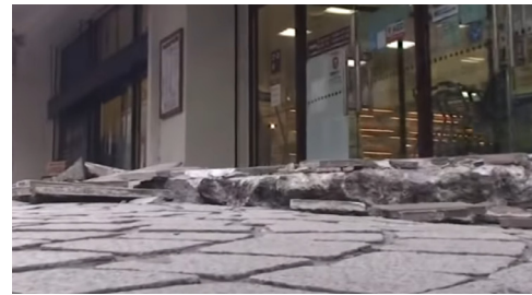
Fig. 8 Separation of the building boundary and ground (containing the boundary-condition nonlinearity) [Video #5]
