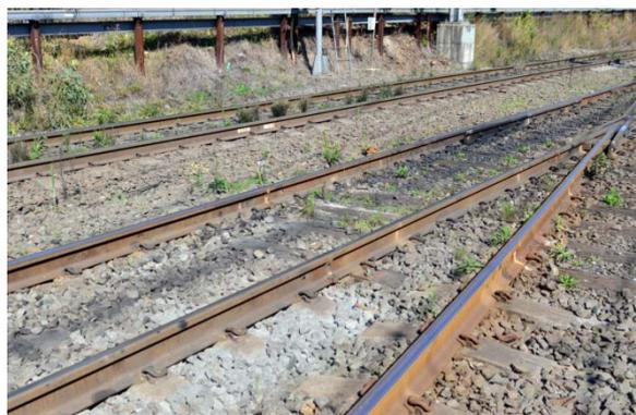
(b) pulverised ballast and track pumping at the interface between timber and concrete sleepers due to the change in track stiffness
