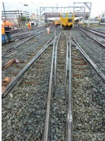
Fig. 9 Double slips installation and resurfacing
