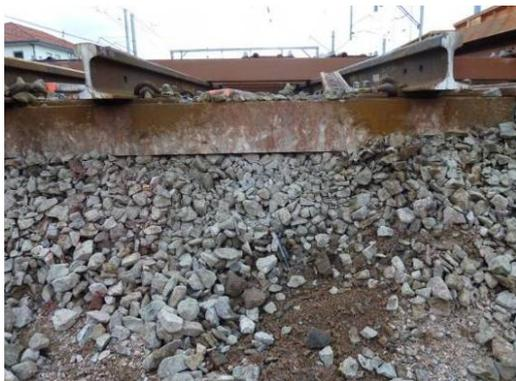
Fig. 7 Cross section at interface between Stages 2 & 3
