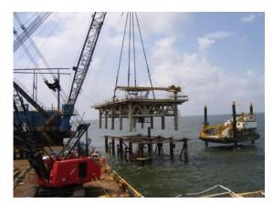
Fig. 1 Decommission of obsolete offshore structure (BSEE 2016)
