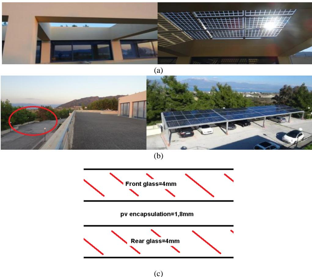
Fig. 3 (a) The skylight before and after the PV installation (Source: authors), (b) The car shelter before and after PV installation (Source: authors) and (c) Project’s PV installation pictures and profile (Source: authors)
