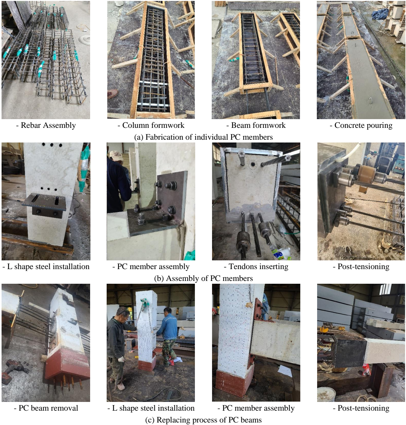
Fig. 4 Manufacturing process of test specimens
