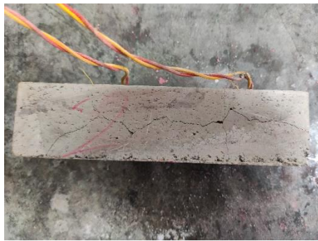
(a) Cracking on tested specimen
