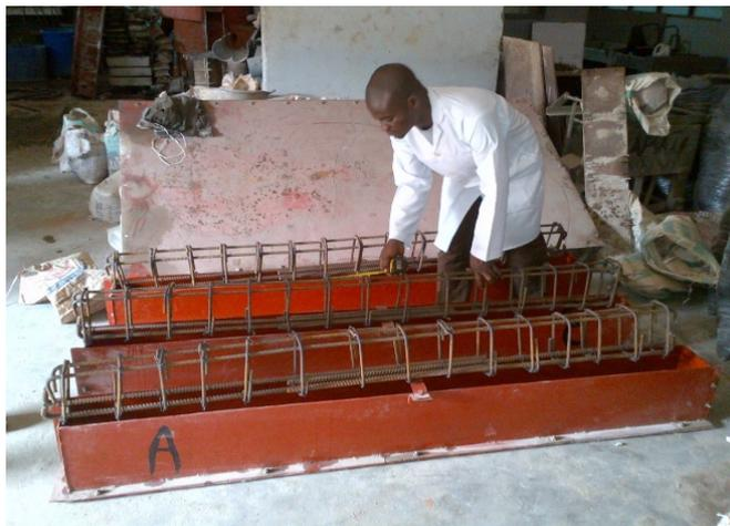
Fig. 2 Reinforcement of spliced beam
