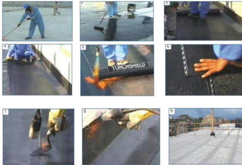
Fig. 1 Waterproofing for roofs with bitumen felt
