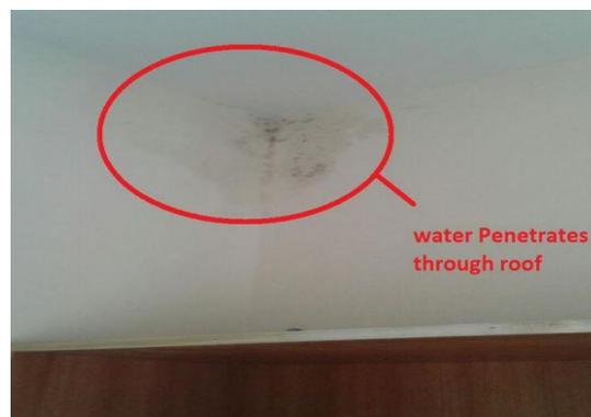
Fig. 8 Water seepage below the roof of slab
