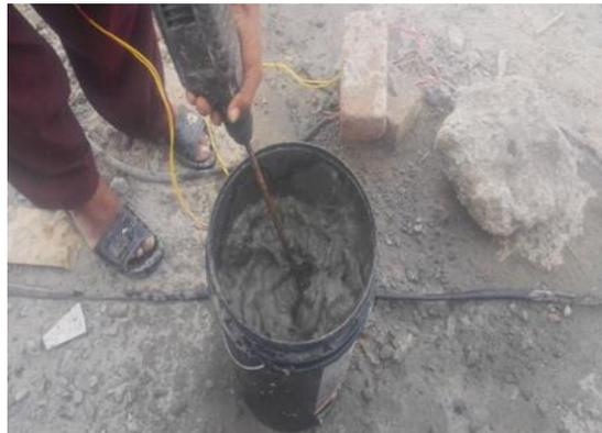
Fig. 2 Mixing of PPPMS slurry with water
