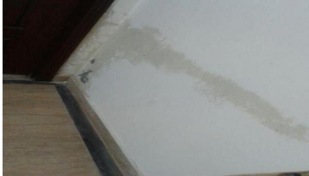
Fig. 9 Seepage on the inner walls of the house due to improper water proofing
