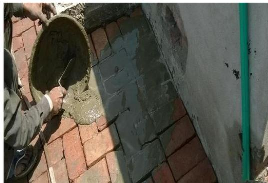
Fig. 7 Smoothing of cement grouting
