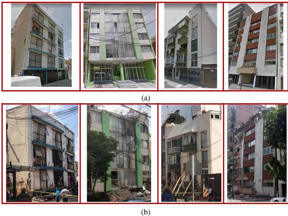
Fig. 5 Collapsed buildings with a soft story - (a) before (Google maps 2017), (b) after (Google maps 2018) the 2017 earthquake
