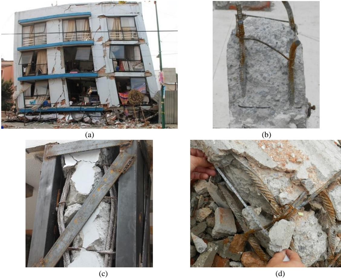
Fig. 1 Typical structural damage - (a) collapsed building, (b-d) damaged columns
