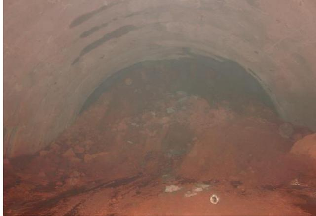
Fig. 7 Collapse situation of the right tunnel
