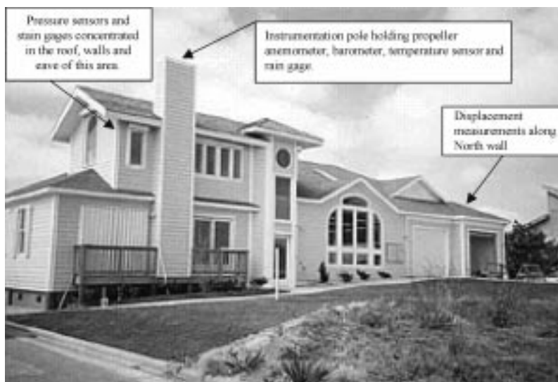
Fig. 1 Front view of the Kern P. Pitts Center before instrumentation was installed. Arrows indicate approximate sensor locations. Note : structure faces east
