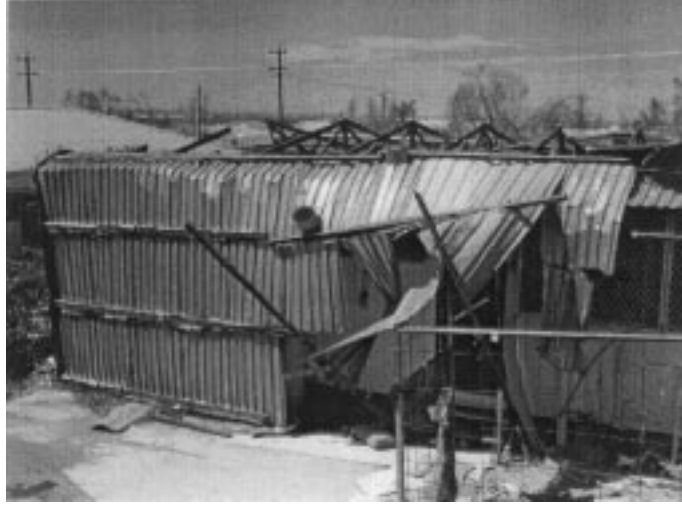
Fig. 2 Failure of roof at the batten-truss connection during cyclone Vance in Exmouth WA.
