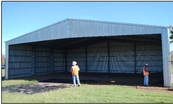
(a) Three-wall shed (gable end wall open)
