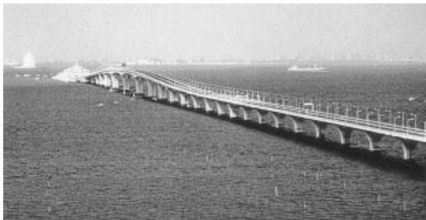
Fig. 1 Box girder bridge where the vortex-induced oscillation was observed during construction
