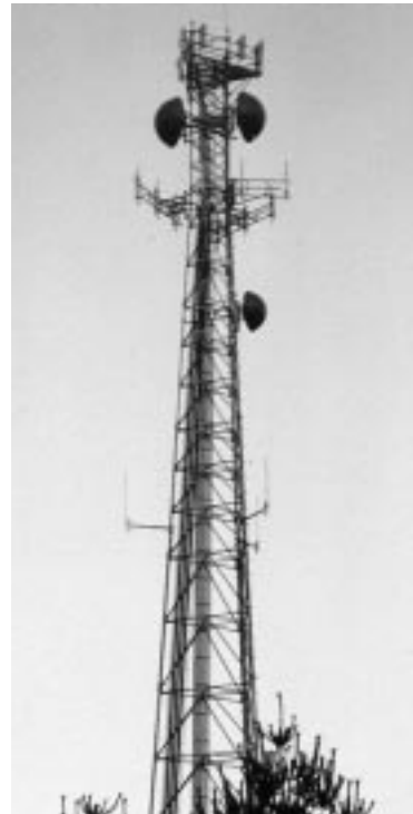
Fig. 2 View of tower with anemometers at 10 m (33 ft) and 57 m (187 ft) heights above ground
