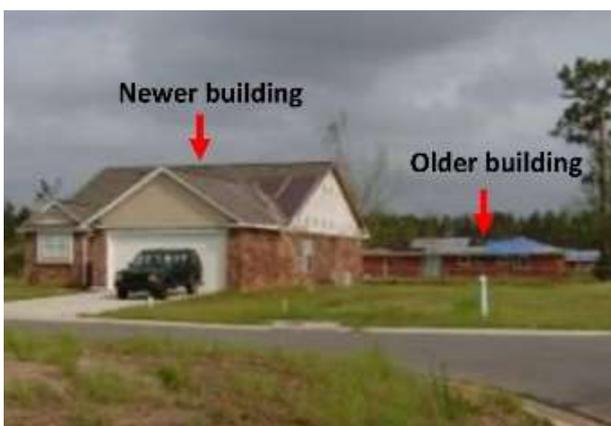
Fig. 1 Newer building with little damage and older building in the same neighborhood with extensive structural damages after Hurricane Katrina (van de Lindt *et al.* 2007)
