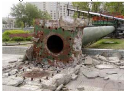
(e) Failure of foundation
