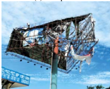
(c) Damage of plate cladding
