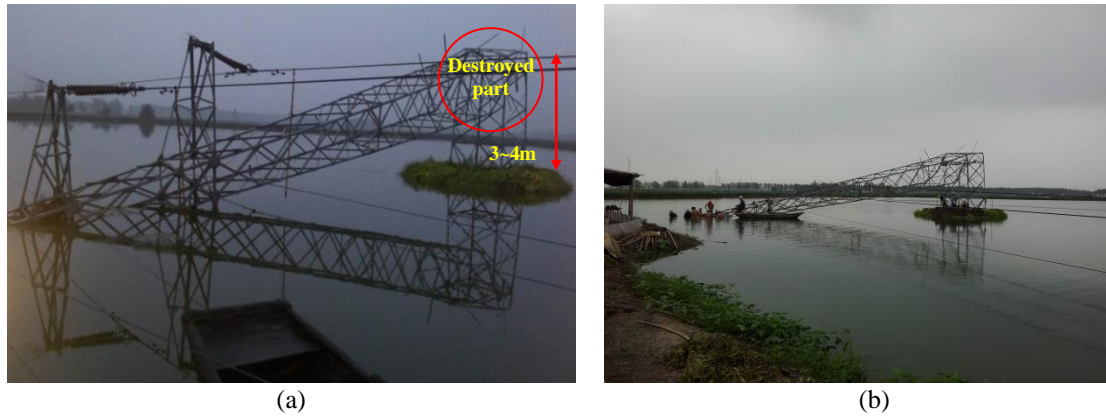
Fig. 4 Collapsed state of the No.18 tower: (a) local view and (b) general view
