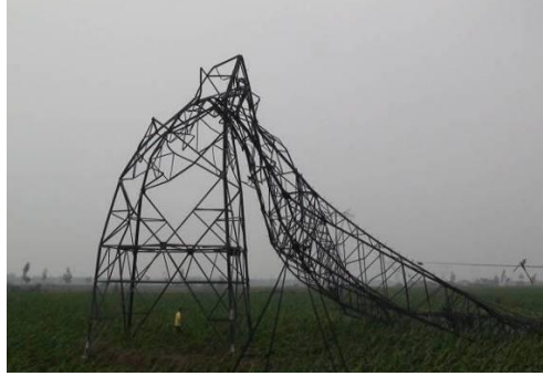
Fig. 1 Failure mode of the typical tower
