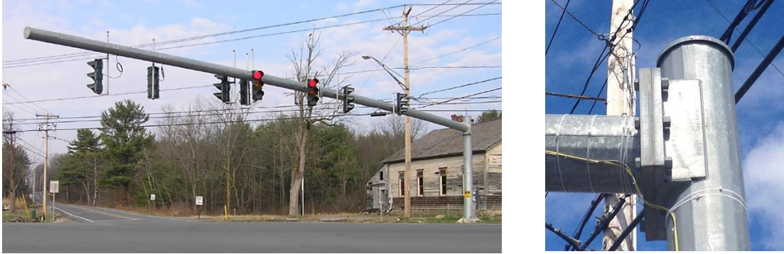
Fig. 1 Mast-Arm Traffic Signal Structure (NYSDOT 2010) (L) and Connection Detail (R)
