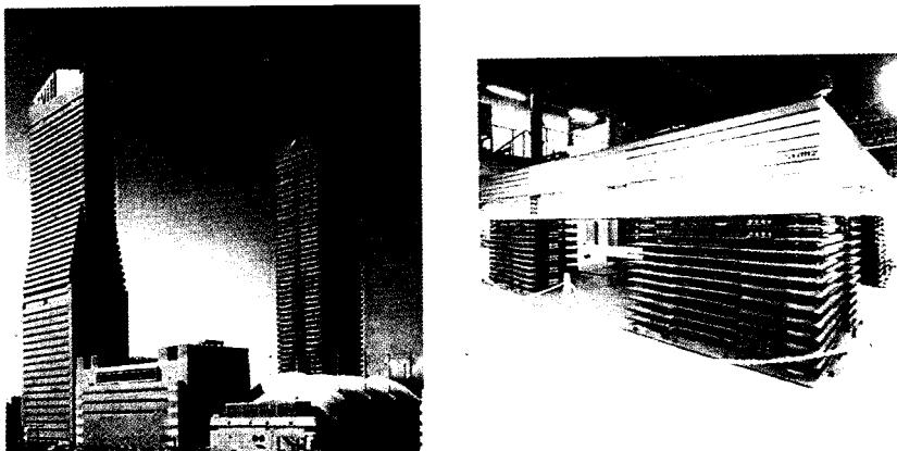
Fig. 23 ORC 200 Symbol Tower and HMD unit installed inside (taken from Yasui Architects & Engineers, Inc.)
