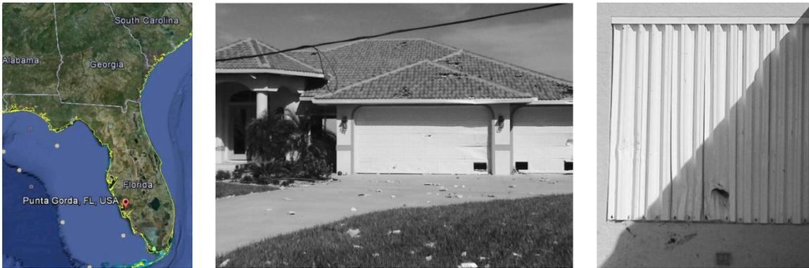
Fig. 1 Tile Debris Damage after Hurricane Charley, Punta Gorda, FL 2004, Left: Map of Punta Gorda, FL (Courtesy of Google Maps), Center and Right: Tile Debris Damage in Punta Gorda, FL
