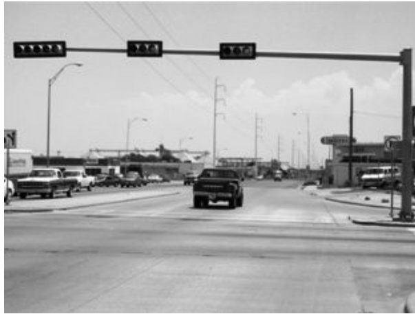
Fig. 1 Cantilever traffic signal structure with straight mast arm
