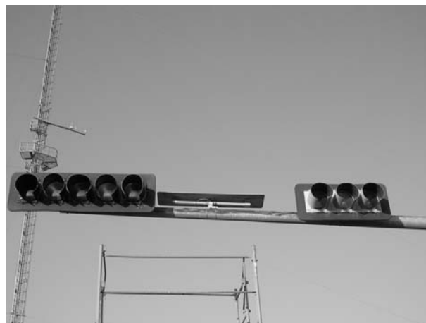
Fig. 21 Mast arm with damping plate
