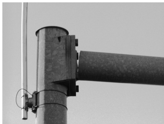
Fig. 2 Fatigue failure of mast arm in Lubbock, Texas
