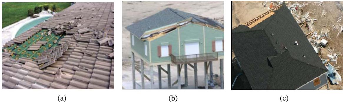
Fig. 1 Damage to roof hip and ridge tiles: (a) Hurricane Charley (FEMA 2005), (b) and (c) Hurricane Ike (IHBS 2009)
