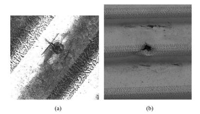
Fig. 1 Cracking patterns following (a) Cyclone 'Tracy' and (b) Cyclone 'Larry'
