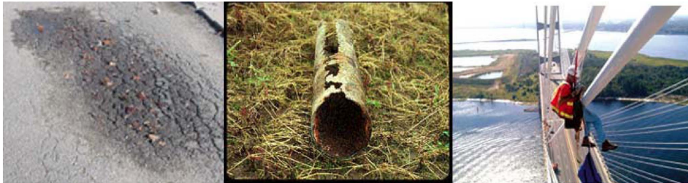
Fig. 1 Examples of moisture-caused infrastructure deterioration: (a) pavement, (b) underground pipe and (c) bridge (stray cable)
