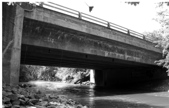
Fig. 6 Photograph of bridge
