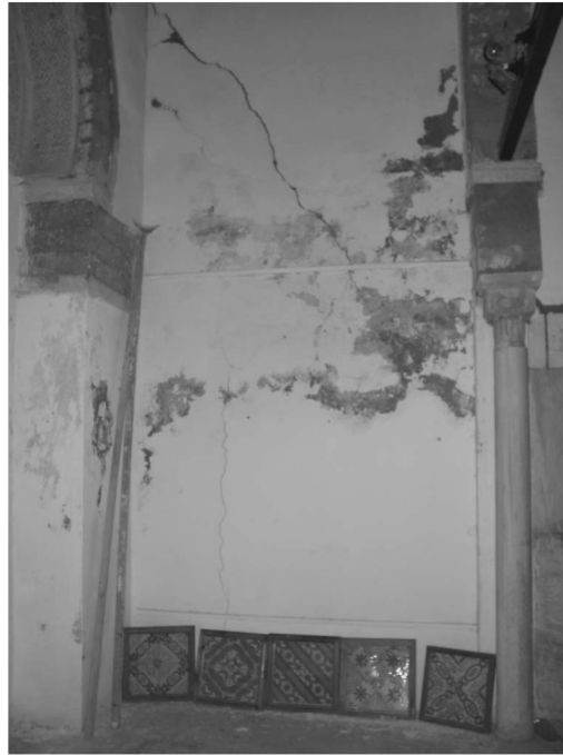
Fig. 2 Cracks in one of the walls of Zaouia of Sidi Kassem Djilizi
