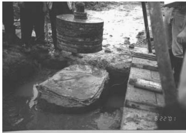
Fig. 5 A lifted weight to be dropped on the pile covered over its head with protection materials
