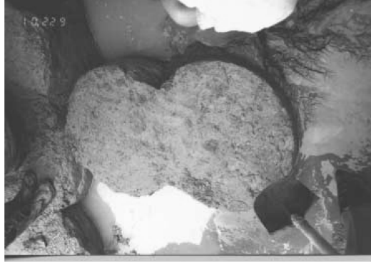
Fig. 1 The cross section of double-head pile for quality evaluation (the diameter of each circular head is 0.7 m and the center-to-center distance of two heads is 0.5 m)
