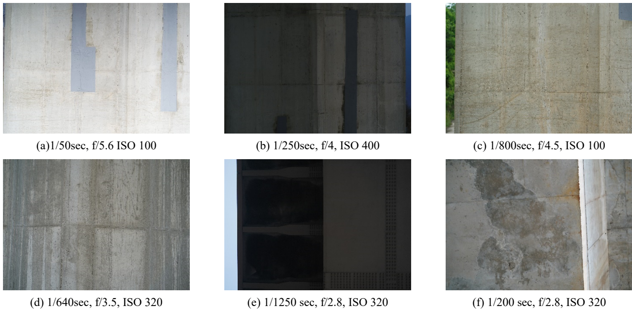
Fig. 3 Examples of obtaining image for bridge inspection using UAV
