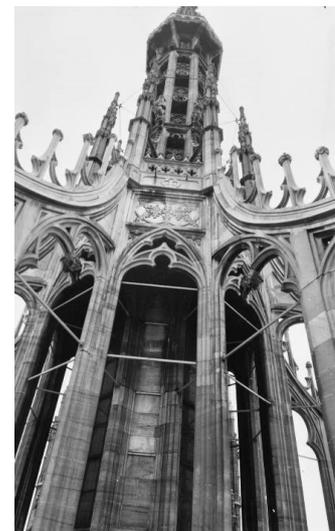
(c) Metallic rods connecting flying buttresses and columns
