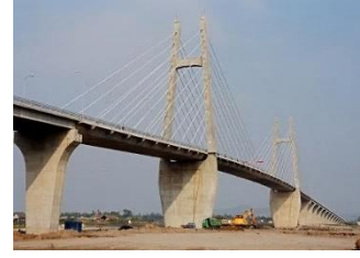
Fig. 3 General view of Kien cable stayed bridge
