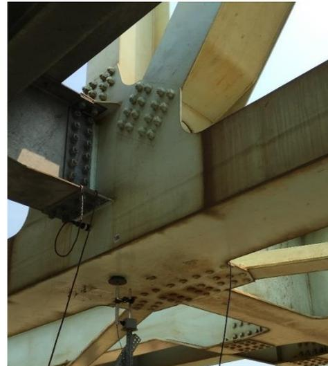
Fig. 7 Placement of accelerometers and LDVTs at one node of Nam O bridge
