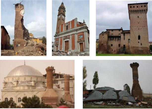
Fig. 1 Photographs of collapsed or heavily damaged historic masonry structures
