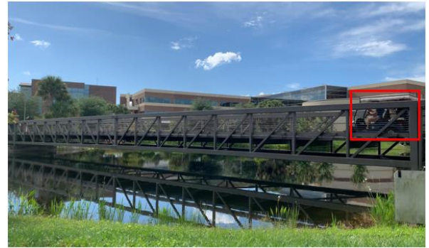
(a) Status of vehicle at the beginning of a truss bridge
