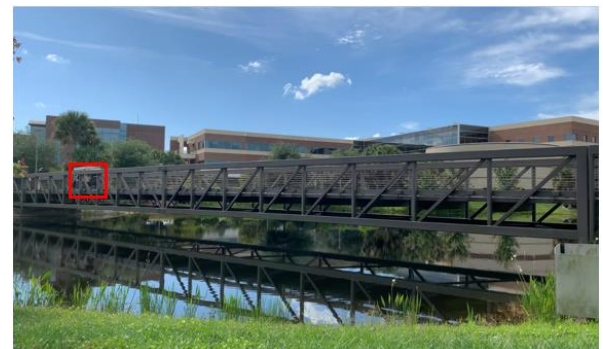
(b) Status of vehicle at the end of a truss bridge
