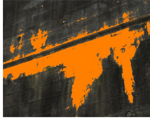
(b) Efflorescence assessment using intensity mimicking visual inspection
