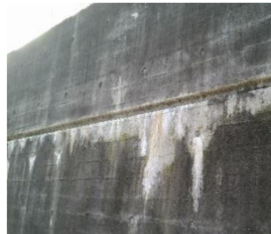
(b) Efflorescence on the north side of the concrete wall (W1-N)
