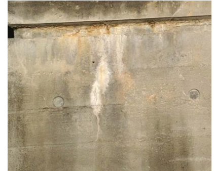
(c) Efflorescence on the west side of the concrete wall (W2-N)
