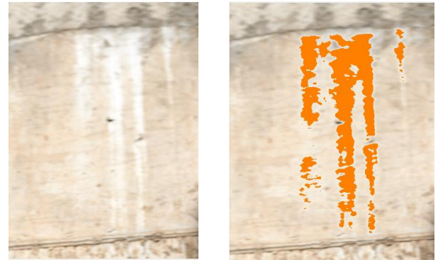
(a) RGB image rebuilt from the hyperspectral image (b) Efflorescence assessment using intensity mimicking visual inspection
