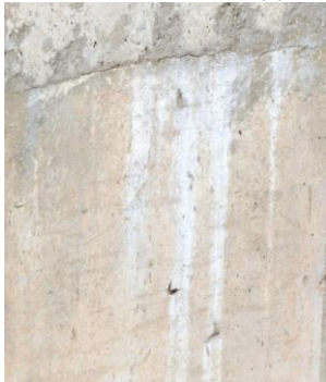
(b) Natural efflorescence on P19 (P1-N)
