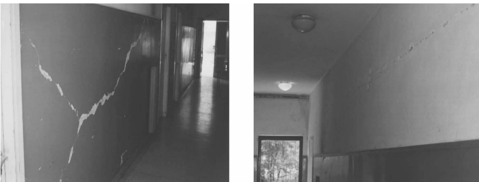
Fig. 2 Wall cracks on the ground floor (left) and infill walls detachment (right)
