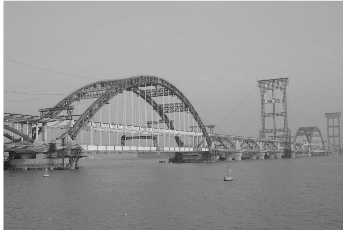
Fig. 4 Picture of QJ 4th Bridge under construction
