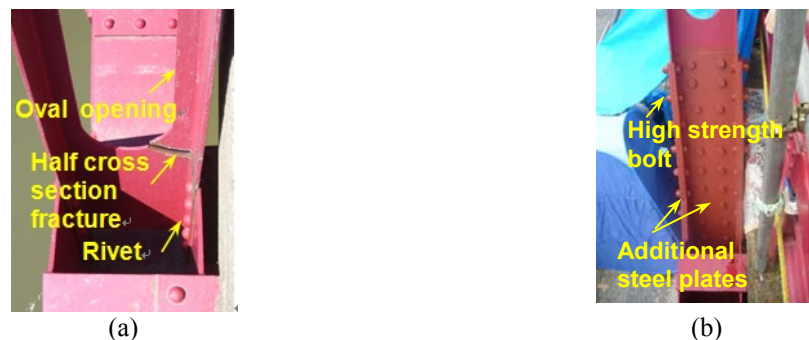
Fig. 2 (a) Partial fracture in D5 in fourth span and (b) repair with additional plates
