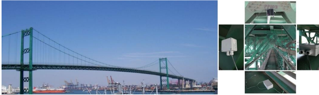
(a) Photo of VTB (left) and installation sensors on the decks and a pipe (right)
